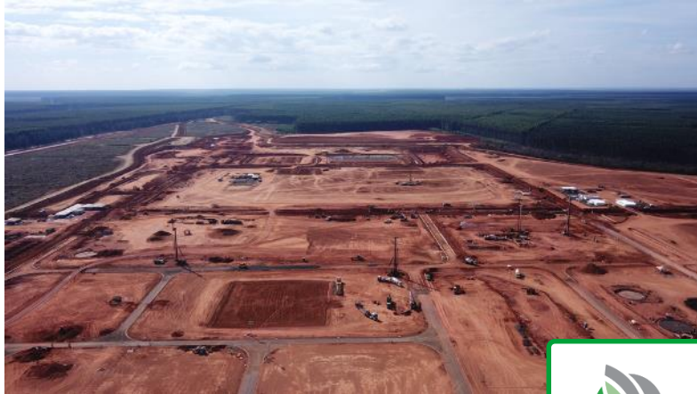
Overview construction site
