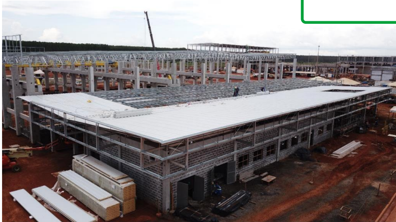
Workshop and Warehouse
