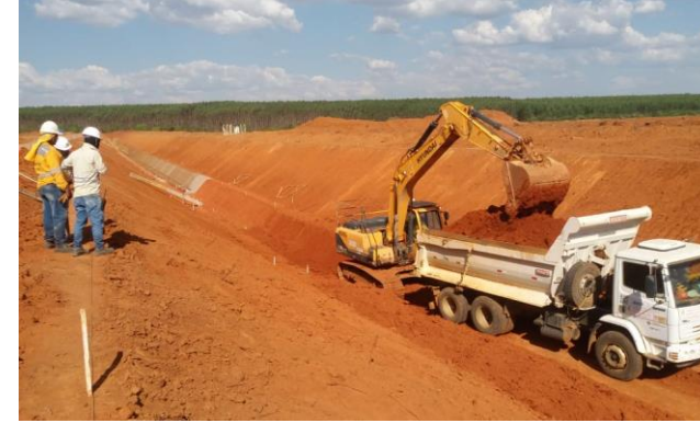
South Channel Excavation
