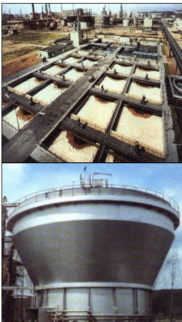
Figure 1. Comparison between flat BOD-plant and the BIOHOCH® reactor.
